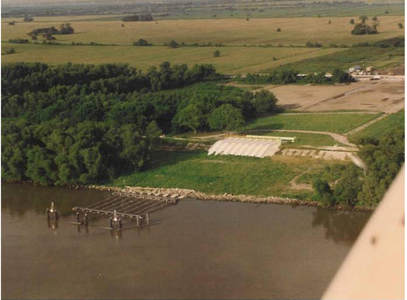
Figure 1. Naomi siphons (BA-03) constructed in 1992 and funded by the State of Louisiana. Mississippi River water is siphoned from the river intakes, discharged into a ponding area and distributed through a single channel into the surrounding marshes.
