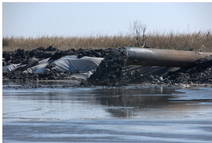
Dredged material from the Calcasieu River Ship Channel is placed in the Cycle III marsh creation site via a temporary pipeline.
