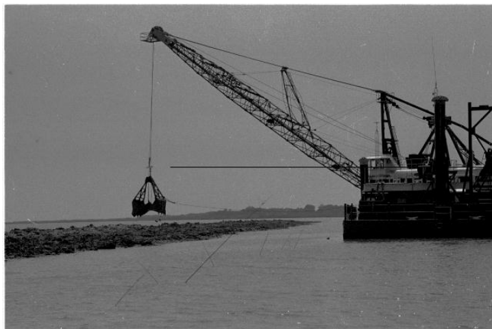
The proposed terraces at Four Mile Canal will be constructed in a similar fashion as shown above. The above photo is of the Captain Buford Berry constructing terraces at the project at Little Vermilion Bay (TV-12).
