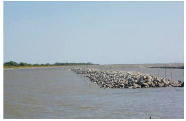
Segmented rock dikes were constructed approximately 200 feet off the shoreline to intercept wave energy before it impacted the beach and caused erosion.
