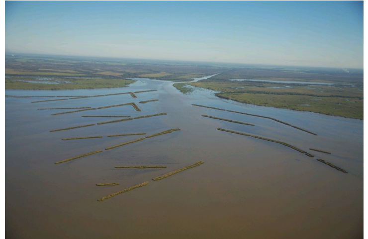
Aerial photo of constructed terraces at the "Jaws" project.
