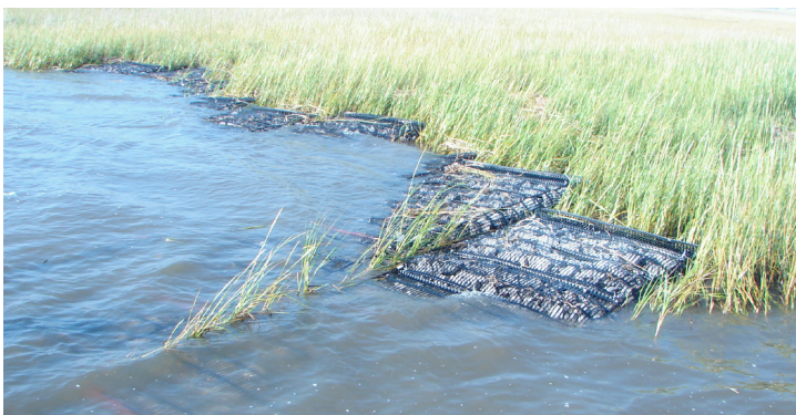
Installed Gabion Mats along the north shore of Lake Barre.
