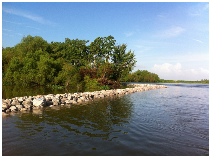
Typical section of forshore rock dike construction as viewed from the GIWW near Copesaw Canal. The typical rock construction includes a lightweight aggregate core to prevent the structure from sinking in these soils that are very organic and have very low load-bearing.
