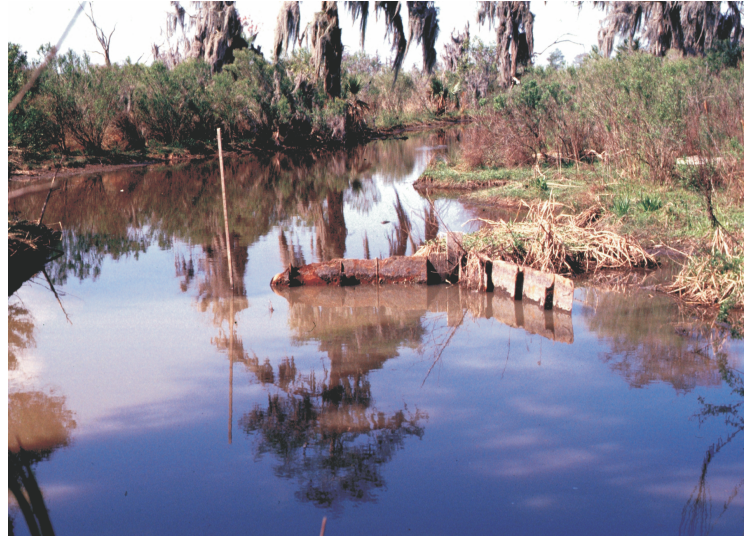
Lapeyrouse Canal will function as one of three freshwater introduction sites along the south rim of Lake De Cade after obstructions are removed and the canal reinforced.
