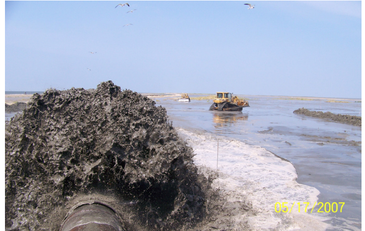
Pumping of dredged sediments on New Cut.
