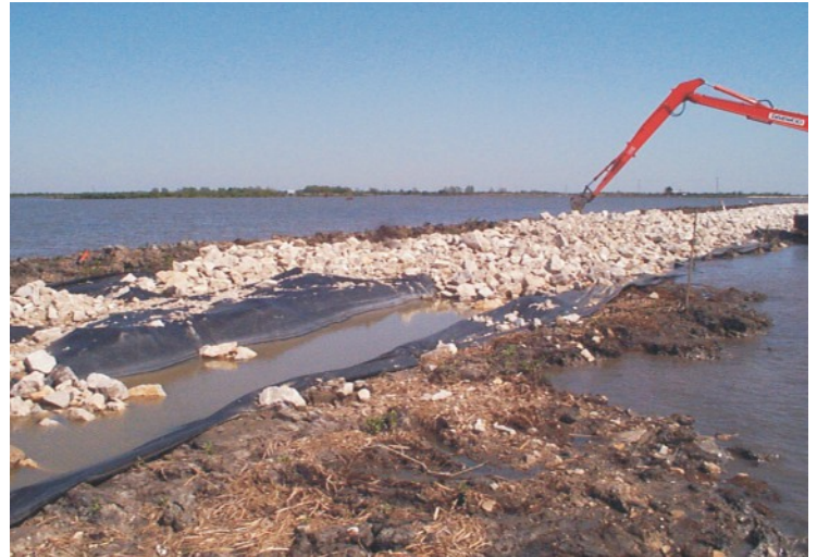
The narrow, eroding shoreline of Bayou DeCade was reinforced with rock in order to help restore the hydrology of the Brady Canal area.
