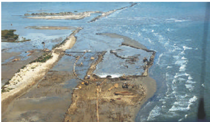
Dredged sediments were pumped onto East Timbalier Island to create a frontal dune system. The Gulf of Mexico is on the right.
