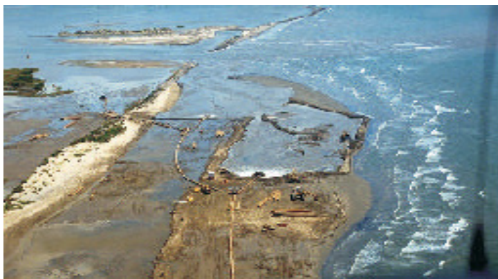
Dredged sediments were pumped onto East Timbalier Island to create a frontal dune system. The Gulf of Mexico is on the right.
