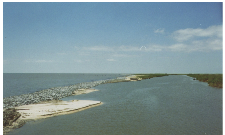
This section of Mobil Canal was backfilled and armored with rock to reestablish the separation between the canal and the gulf so that salt water would be prevented from damaging the intermediate marshes in the interior of the island.
