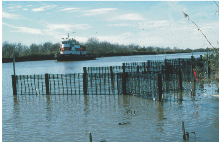
One of the six types of wave-damping structures tested for their ability to protect the canal's shoreline.
