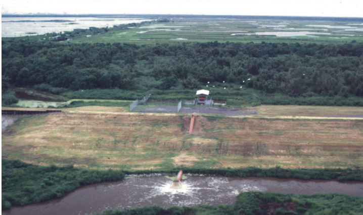
A Bayou Sauvage pump station in operation, facing west. It is removing water from the project area, depicted in the upper portion of the image.
