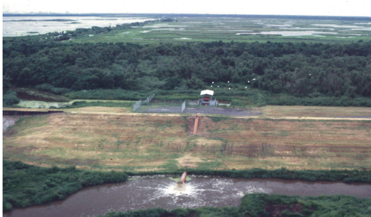
A Bayou Sauvage pump station in operation, facing west. It is removing water from the project area, depicted in the upper portion of the image.
