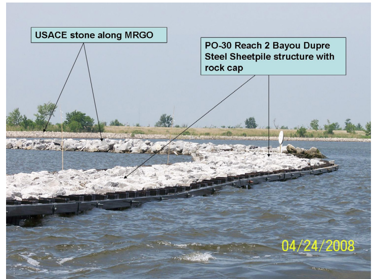
Double wall steel sheet pile structure at Bayou Dupre.
