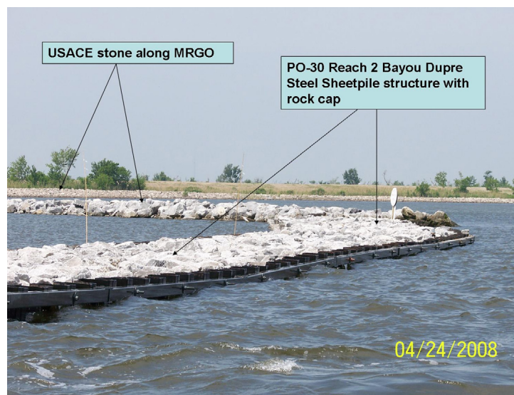
Double wall steel sheet pile structure at Bayou Dupre.
