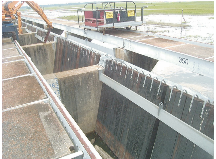
The Bonnet Carre Spillway timber pins will be pulled for opportunistic use of the structure.
