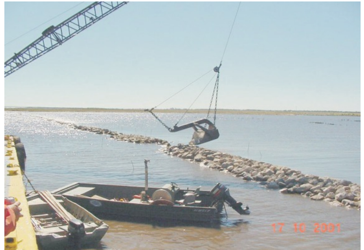
Rock being placed at Bayou Chevee.
