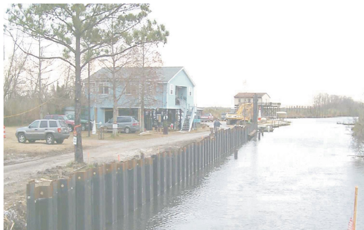
Steel sheet-pile will ensure that erosion will not enlarge this cross-sectional area of the channel. Actions such as these will restore a more natural hydrologic regime to the area.
