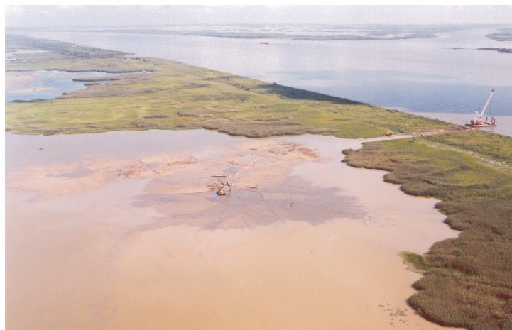
View of marsh creation area during placement of dredged material.
