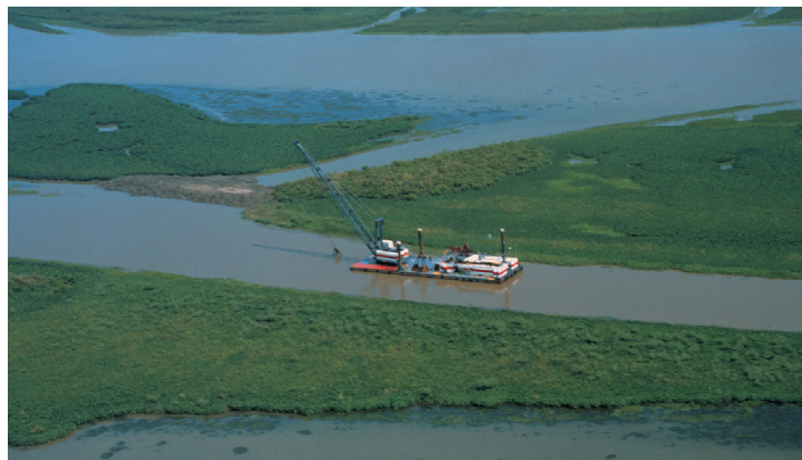
This image shows a crevasse being plugged in 1999 in order to maximize the effectiveness of crevasses downstream. As this project contains several building cycles, project components are adjusted over time to achieve optimal performance as new features are constructed.
