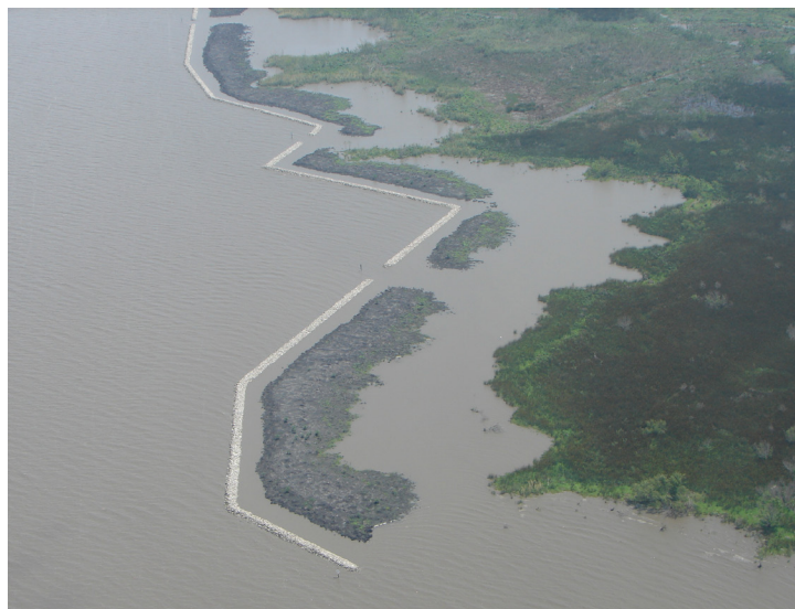
Segmented rock breakwaters such as the one constructed above will provide protection for White Lake's eroding shoreline.
