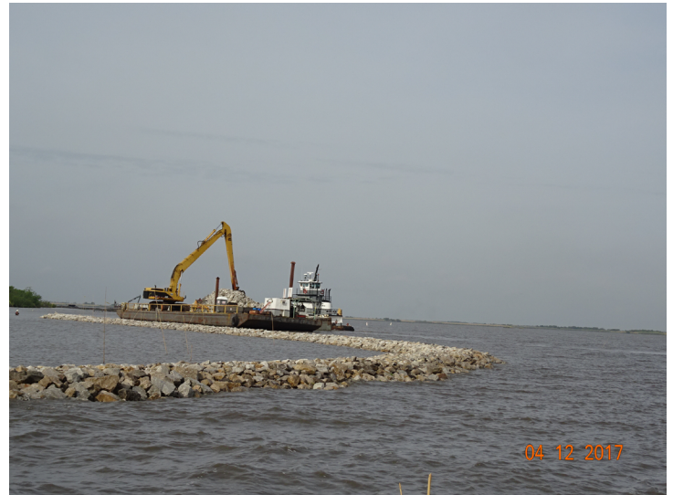
Construction of the project's stone breakwater.
