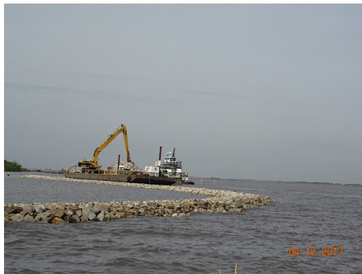
Construction of the project's stone breakwater.
