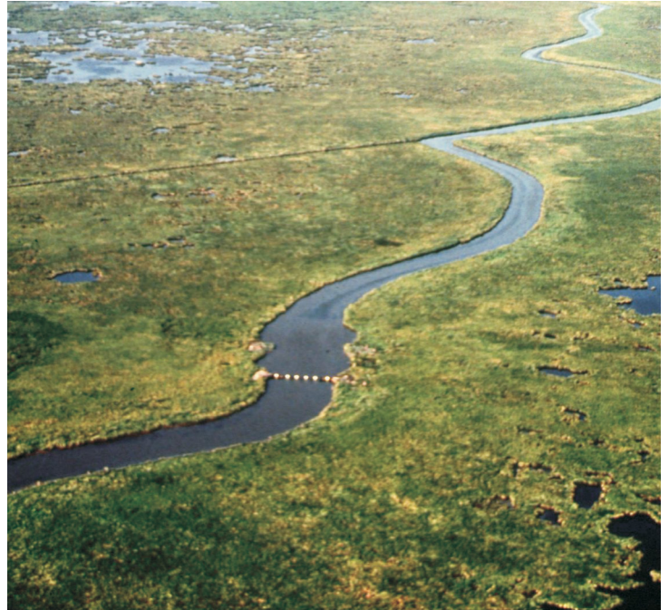
Perimeter structures, such as the one shown above, and other project features will be used to restore hydrology in the project area.
