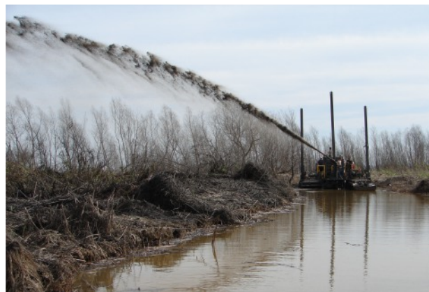
Small spray dredge enlarging the Grand Volle Ditch and spraying the spoil over existing marsh.
