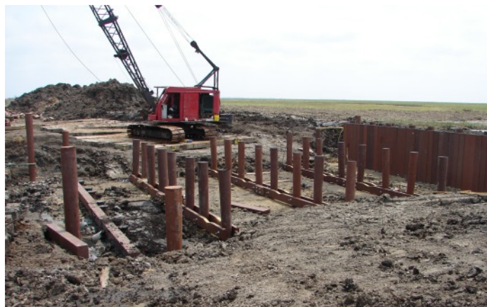
Early stages of the construction of a water control structure to move freshwater to brackish marshes to the south.
