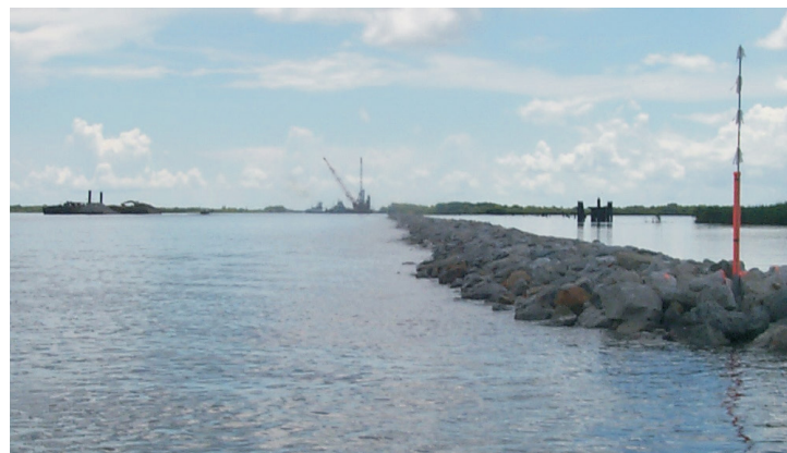
This continuous rock dike will drastically reduce boat wake-induced shoreline erosion.
