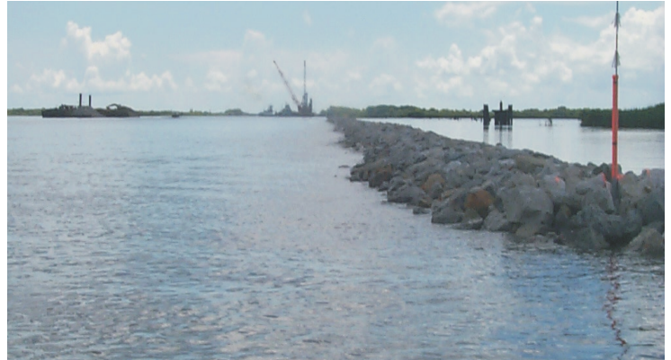
This continuous rock dike will drastically reduce boat wake-induced shoreline erosion.
