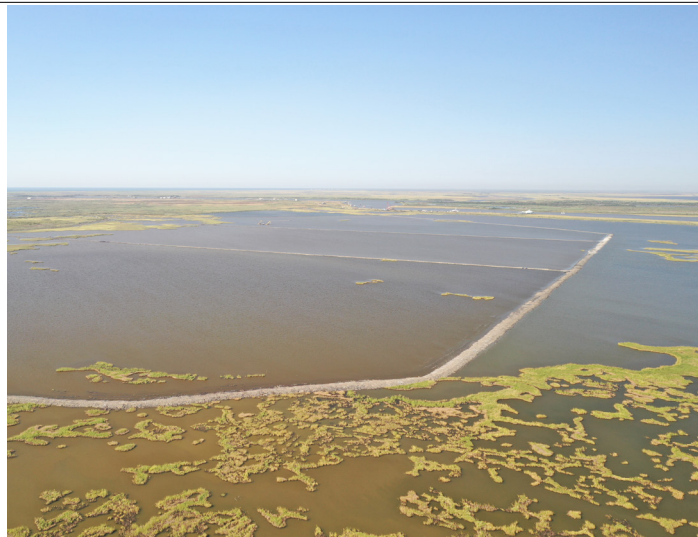
Photograph of the external and internal containment dike construction progress of the No Name Bayou Marsh Creation and Nourishment project.
