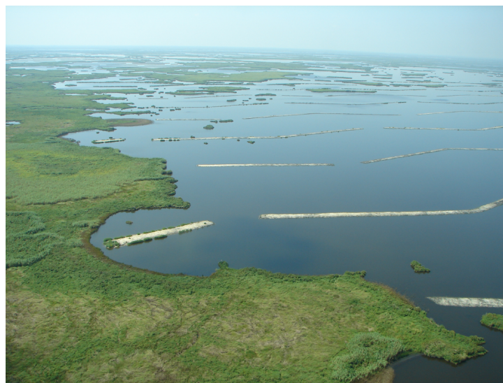
Portion of the 232,000 linear feet of vegetated earthen terraces constructed near Greens Lake on Sabine National Wildlife Refuge.
