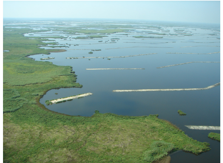
Portion of the 232,000 linear feet of vegetated earthen terraces constructed near Greens Lake on Sabine National Wildlife Refuge.
