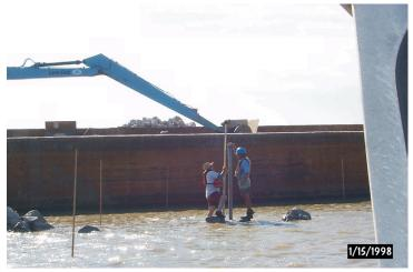
Settlement plates such as the one pictured here will be used to determine if settling of the structure has occurred. Technicians from NRCS's Crowley Watershed Office are shown taking baseline elevations before more rock is deposited. Future elevation readings will be taken after the structure is completed.
