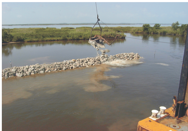
Above is the rock dike under construction. A large open water area is in the background.
