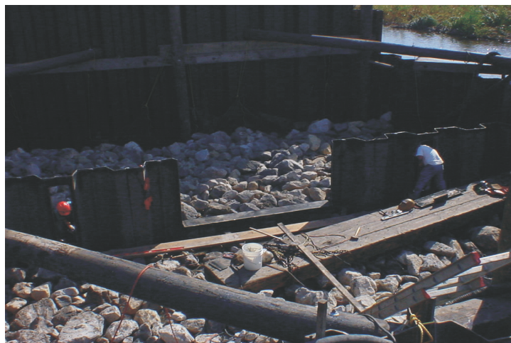
This picture was taken during installation of the self-regulating tidegate (SRT). Fish slots on either side of the SRT will allow movement of marine life between the areas when the gate is closed.
