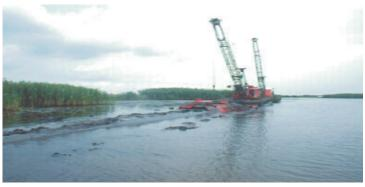
Even though two large pieces of equipment were required to tow the plow through the water, efforts during project implementation showed this method to be less time consuming than utilizing traditional equipment such as a bucket-type dragline.
