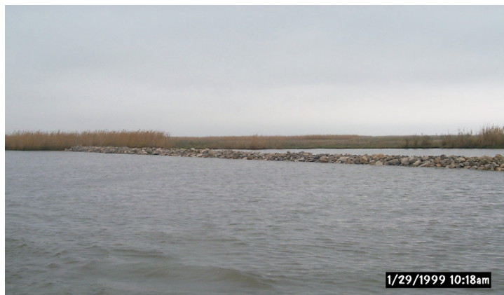
Rock riprap which can withstand the destructive forces of wave energy helps to maintain the integrity of the shoreline.
