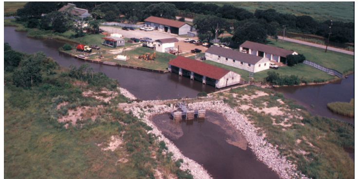
The Sabine National Wildlife Refuge's new Headquarters Canal water control structure (looking southwest) is comprised of three 5-ft diameter culverts with sluice and flap gates. The refuge headquarters buildings are in the background, and LA Hwy 27 is to the right.
