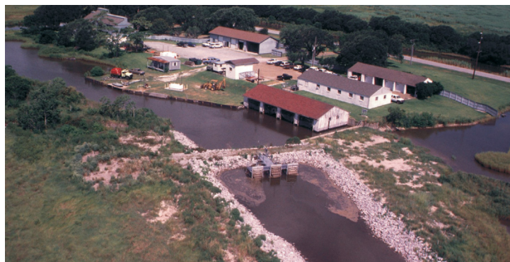
The Sabine National Wildlife Refuge's new Headquarters Canal water control structure (looking southwest) is comprised of three 5-ft diameter culverts with sluice and flap gates. The refuge headquarters buildings are in the background, and LA Hwy 27 is to the right.
