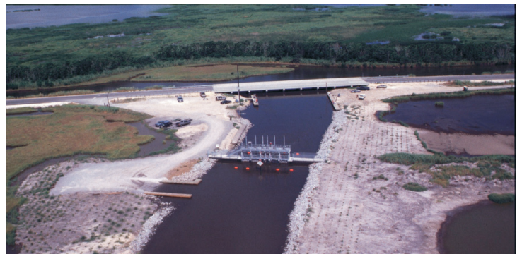
Looking west at the Hog Island Gully water control structure on the Sabine National Wildlife Refuge. The structure has four large 7.5-ft wide by 8-ft deep bays and two smaller 3.5-ft wide by 8-ft deep bays with slide gates. LA Hwy 27 is in the background. The West Cove structure is similar, but with three bays instead of four.
