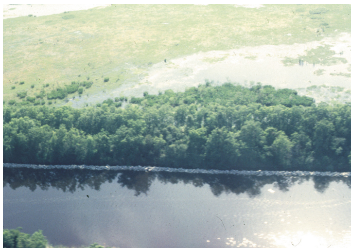
Sabine National Wildlife Refuge Erosion Protection looking eastward across the Burton-Sutton Canal into Pool 3. The continuous rock breakwater is seen along the shoreline in the lower third of the photo.
