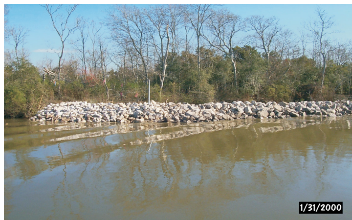
In order to prevent the GIWW from encroaching into the lakes, the thin, eroding shorelines were protected with rock riprap.
