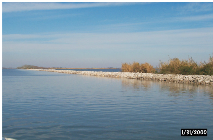
In some areas, the shoreline was non-existent, succumbing to the forces of wave erosion. A new barrier consisting of rock was constructed, ensuring a more natural water flow in the project area.
