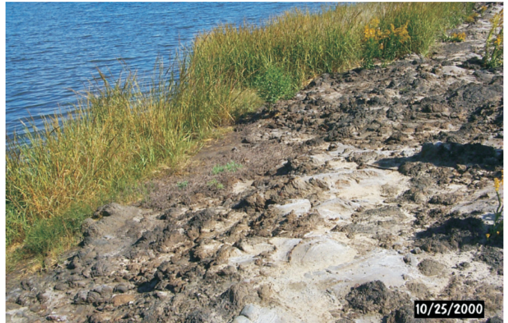
In order to prevent wind generated wave erosion from destroying the freshly added spoil, vegetation is planted to get a head start on providing cover for the fragile soil.
