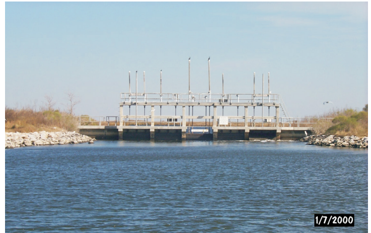
Structures such as this one help regulate the amount of salt water that enters the marsh, improving the health of wetland vegetation.
