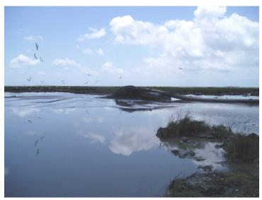
This 24-inch dredge pipe is actively rebuilding marsh by depositing sediment dredged from the lake. As the project progresses, the placed sediment will reach an elevation conducive for growing and sustaining marsh vegetation.
