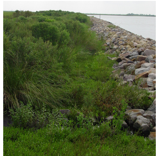
This photo illustrates the rock revetment protecting the vegetative shoreline.
