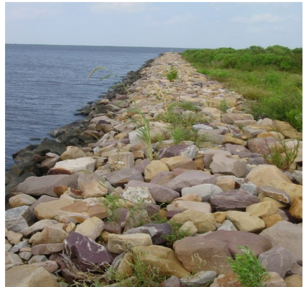
Five years after construction, the constructed rock revetment has proven to be very effective at eliminating shoreline erosion.
