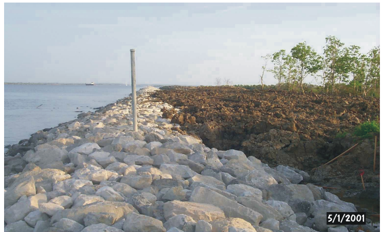
This completed rock riprap structure was placed adjacent to the existing shoreline to buffer it from the erosive forces of wake-induced wave energy.
