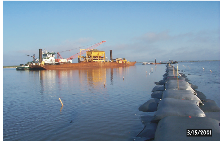
Geo-textile fabric bags were filled with a lightweight aggregate and then sewn closed. These bags act as the supporting core of the shoreline stabilization structure.
