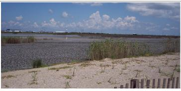
Dredged material from the Gulf of Mexico was pumped into the project area to create and nourish approximately 900 acres of back barrier marsh. This project works synergistically with the state-led Caminada Headland Beach and Dune projects (BA-45 and BA-143), constructed in 2015 and 2016. Photo credit: EPA, May 2023.
