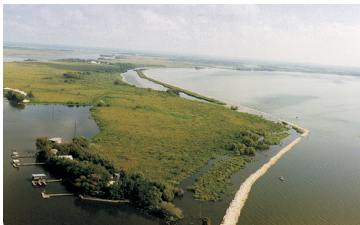
Phase 2 of the Lake Salvador restoration project. The rock structure shown was installed to help stabilize the shoreline, allow sediment trapping, and promote marsh development.
