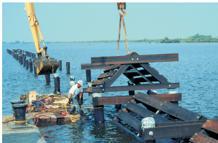
Installation of an erosion control structure during Phase 1 of the Lake Salvador restoration project.
