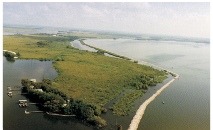
Phase 2 of the Lake Salvador restoration project. The rock structure shown was installed to help stabilize the shoreline, allow sediment trapping, and promote marsh development.
