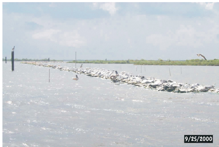
The constructed rock breakwater located in Bay L'Ours will assist in reducing wave energies before they impact the shore and will also arouse the curiosity of local waterfowl such as these pelicans.
