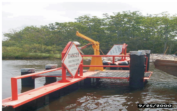
This winch which is permanently attached to the variable crest, water control structure located right off Briton Canal, will help to configure the structure according to a pre-determined water management plan.
