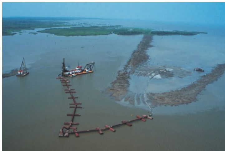
A hydraulic dredge pumps sediment to create new wetland habitat in the project area south of Morgan City.
