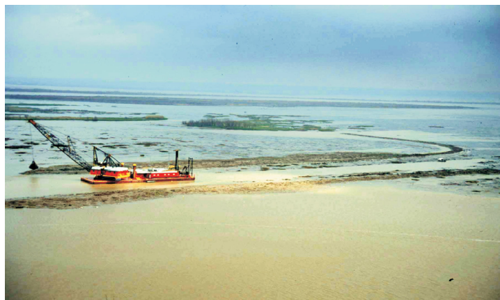
A bucket dredge is shown removing sediment from a shoaled-in channel in order to help reestablish water and sediment flow within the Atchafalaya Delta.
