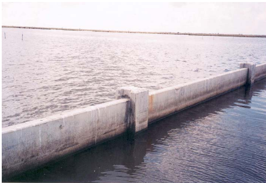
Figure 4A: Concrete pile structure, constructed as part of Construction Unit 1 in April-May 2001.
